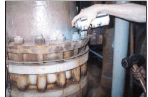
Two men easily remove flange bolts in 2 hours with Chesterton 723 Sprasolvo®.
