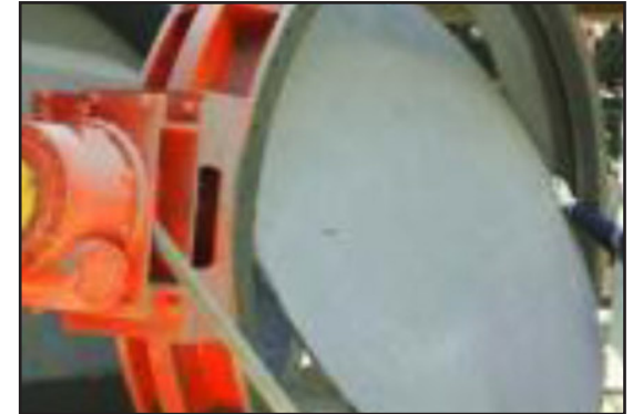
Completed valve with ARC S4+ topcoat applied
