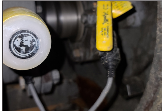
Chesterton Connect sensor installed in pump.
