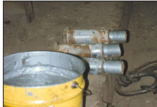
New hinge bolts and nuts are coated with Chesterton 725 Nickel Anti-Seize.
