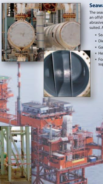
The erosive and highly corrosive fluids commonly found inside production equipment on offshore production platforms are areas where ARC Composites are providing years of reliable service. Examples where ARC Composites are providing extended service life for production-associated equipment include internal linings of:
