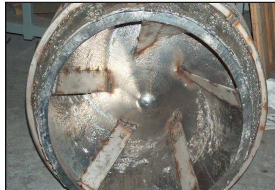
Weld repairs to the impeller vanes
