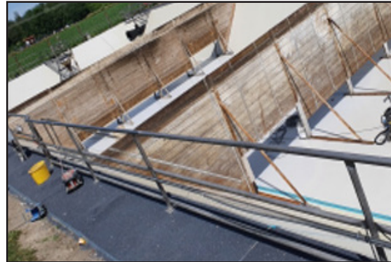
On-going application of ARC CS2(E) in one of the tanks.
