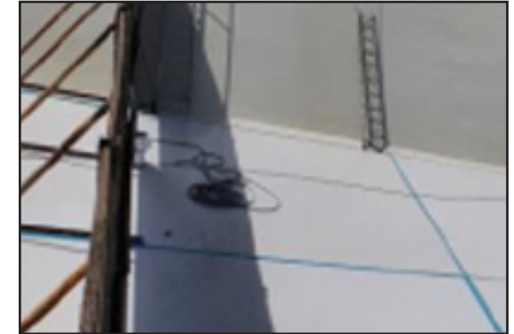
Result of the renovation with ARC CS2(E) .
