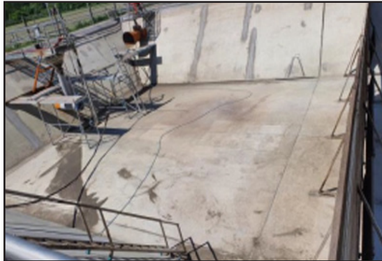
Aeration tank before renovation.
