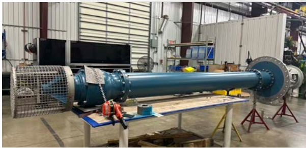
VS1 Vertical Turbine Pump Repair
