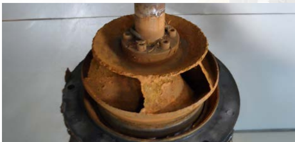
Before – Repair of Pump with ARC Composite Coatings
