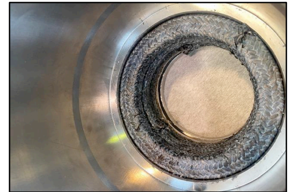
Chesterton 377 CarbMax Packing installed in stuffing box.
