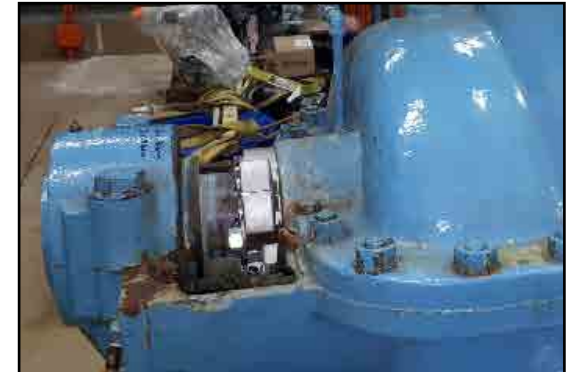
The 442C Split Seal completed installation.
