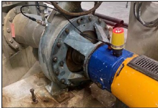
Chesterton Connect Sensor monitoring discharge pressure and bearing temperature.
