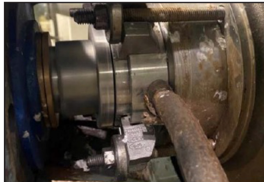
Chesterton 1510 Cartridge Seal installed on a centrifugal pump.
